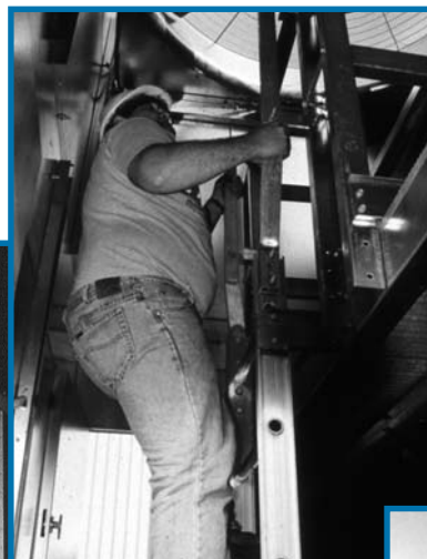
Internal service platform with ladder
